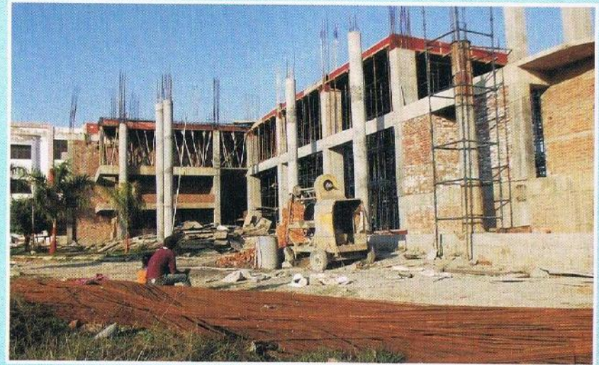
Multipurpose Sports Complex & Auditorium Work in Progress
